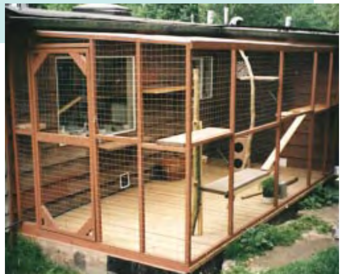
Simple kitty house, coarse mesh hardware cloth on 2x2s with shelves and ramps. British Columbia
